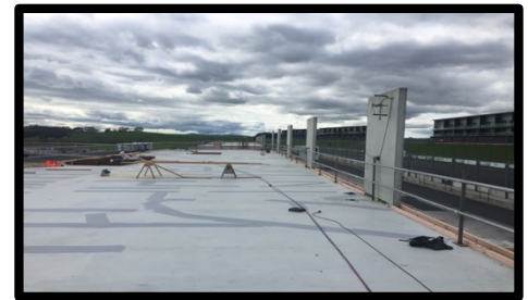
On top of existing pit lane structure
