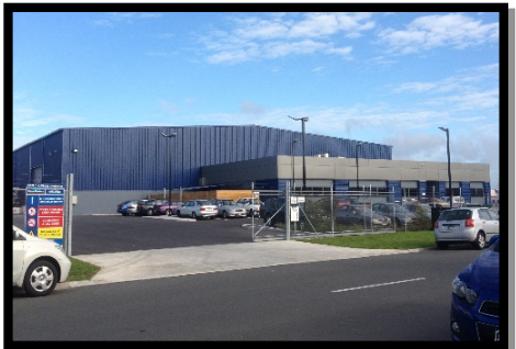
Placemakers frame and truss plant
