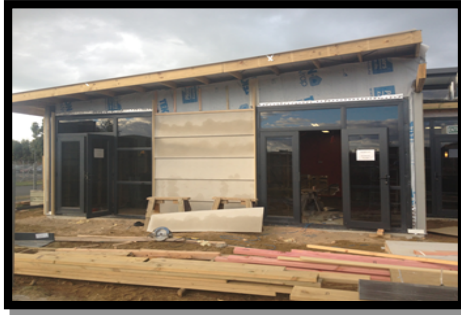
Dairy goat co-op office renovation
