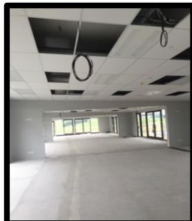
Photo taken during construction showing floor leveling compound that has been laid and suspended ceiling grid going in.
