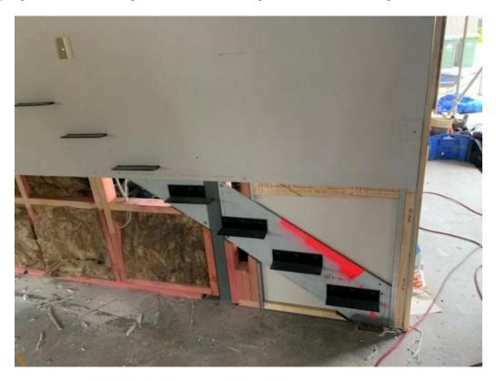
To start, we worked out what the height from the finished floor level was, how far it was going to go and then calculated the ride and run for every step. We started by marking out where our steel plate would be fixed to the wall, from top to bottom. We checked out the exact depth of the steel into the framing to ensure the Gib would float over the stringer in a way that no one would know it was there (as seen in the photo beside).
