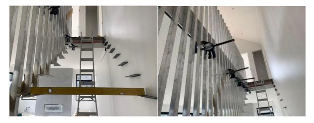
Due to the size and weight of the balustrade, it was broken up into two parts and then bolted back together into the mid floor on site. I then set out the building of the stairs. We received each step individually (one rise/run).
