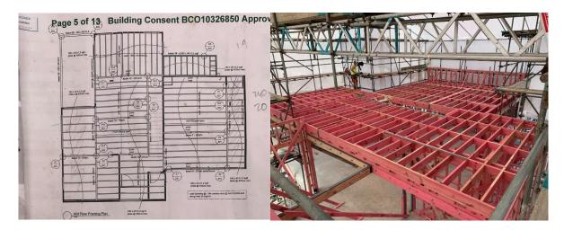
The roof framing of the second storey was one of my favourite elements of this build. Two gables side-by-side with an internal gutter and a mix between rafters and trusses provided me with plenty of learning opportunities. Both gables were pitched at 35 degrees and we built the frames ourselves. This meant we had the opportunity to draw the frame out on the floor to the exact measurements and build the gable ends to suit.
