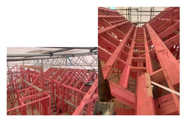
I was excited by the challenge of framing up the internal gutter. The minimum fall was 1 in 100 with the smallest flat section being a minimum of 350mm. As you can see from the framing photos above, it perfectly copies the plan. I particularly enjoyed framing up this section of the roof as it was something I hadn't previously done so to tick off an internal gutter was exciting. The gutter was lined with 19mm H3.2 plywood and then the water proofers came and completed the waterproof membrane.
