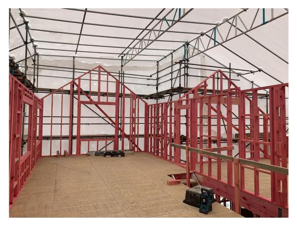
This project incorporated a combination of rafter and trusses, dictated by the ceiling design. The rafters provided a raking ceiling, and the trusses were used for flat ceilings.
