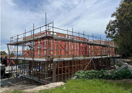
first floor frames we had a large focus around our lift shaft and stair well. We wanted to make sure that these frames were put in perfectly plumb from the top plate of the first floor all the way down to the bottom plate of the ground floor. We were able to use a weighted plumb bob to determine the exact position of our first floor frames. By getting these plumb at this stage of the build it was able to speed us up massively when we came to straighten the inside of these areas.
