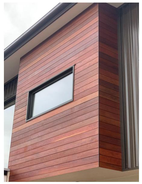
that we put them in plumb, straight and parallel so we could cut all our LMA boards to the same length from top to bottom. We also installed j mold flashings on each side of every window and all internal corners. These would not be seen but were required for waterproofing.
