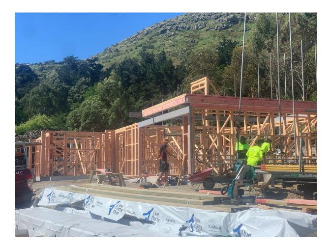
Our next job was to connect our frames and steel together as seen in the photo to then right. We did this by bolting timber to the side of the steel and then framing it out to make it one solid structure. We also put timber infills inside of our steel columns to make sure we had fixing and the correct overhangs as per plan. After plumbing and straightening everywhere the steel
