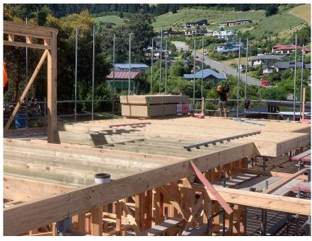
were then able to quickly cut the rest of the sg8 joists to length and nail them flush with the top of the lvl beams. Doing it this way helped speed up the process immensely. We then quickly checked over our work with a big straight end and buzzed down any high points. This ensured our floor would be perfectly straight.
