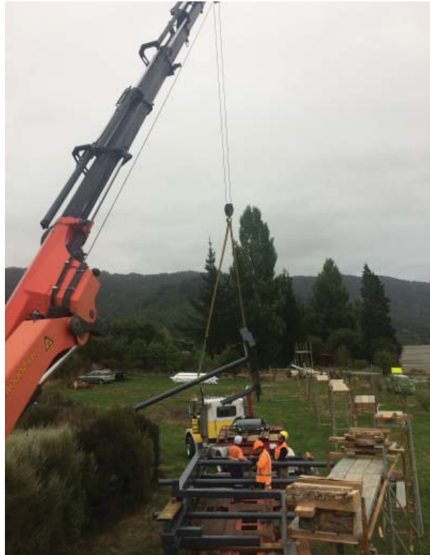
Fig. 19: Temporary scaffolding is set up for each module.
