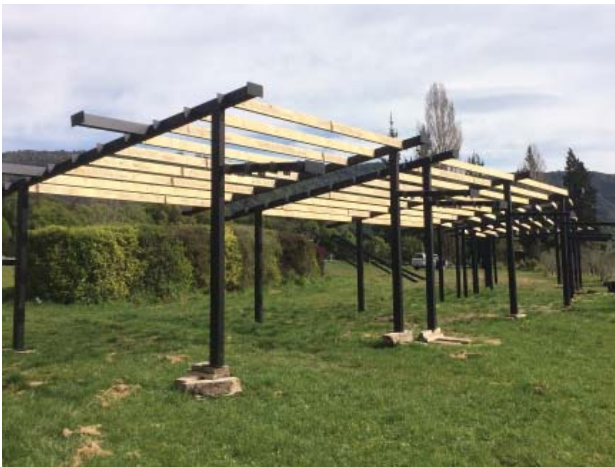
Fig. 51: Four legged modules created by bolting 150x50 Hyspan rafters between two steel portal frames.
