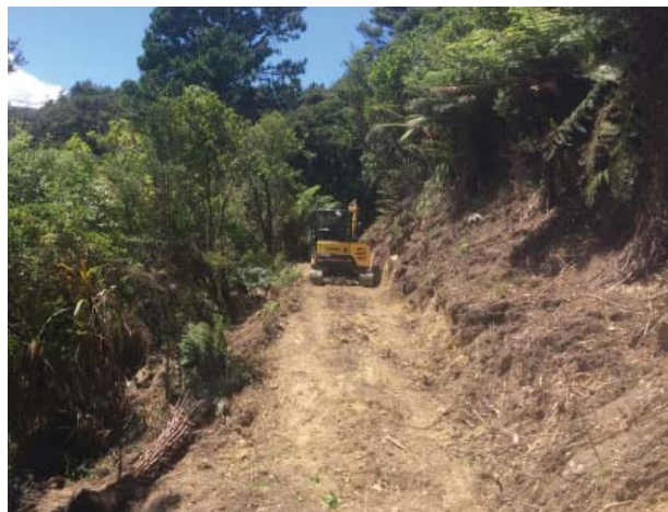
Fig. 11: Benched track to access pile locations above and below.
