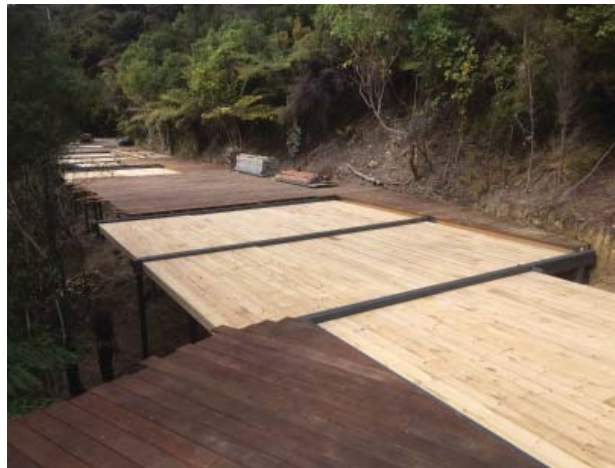
Fig. 45: C.L.T panels act as a diaphragm providing horizontal bracing. Panels are fixed to steel bearers with 200mm coach bolts at 600 centres.
