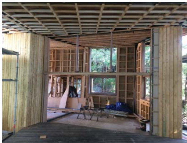
Fig. 91: Weatherboards are 4600mm long in some places.
