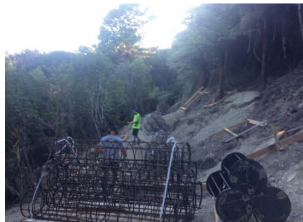
Fig. 17: Rebar cages on the left, and pile caps on the right.
