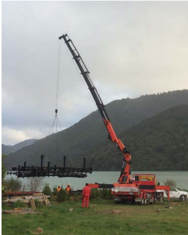
Fig. 49: Portal frames arriving at David's yard for prefabrication.
