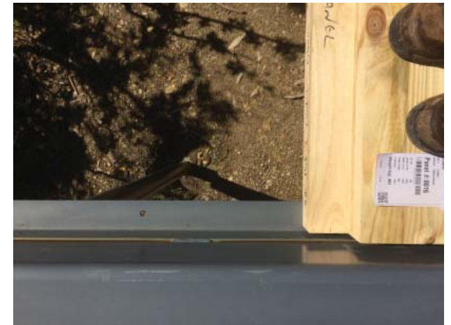
Fig. 46: Where C.L.T panels join they overlap one another. There is 10mm tolerance between steel bearer and C.L.T panel.
