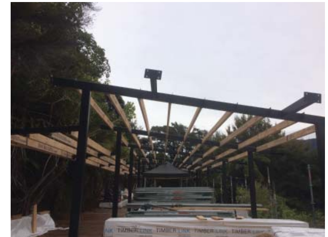
Fig. 53: Modules delivered on site. Steel outriggers will pick up flying rafters to create eaves.
