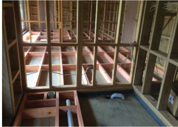
Fig. 93: Pre-wire and pipe out is underway
