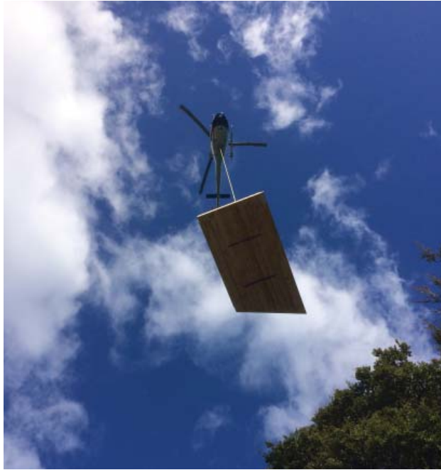
Fig. 41: Helicopter delivering a Cross Laminated Timber (C.L.T) panel.
