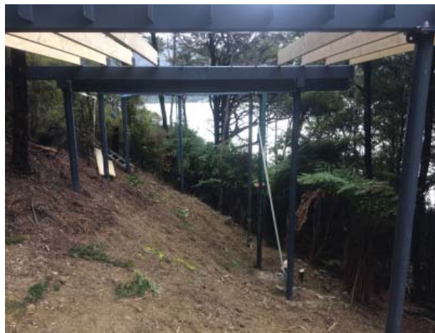
Fig. 27: Deck joists bolt efficiently to cleats on the portal frames.
