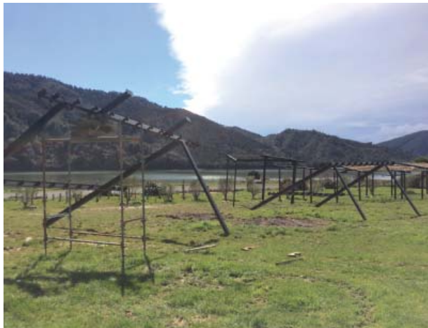
Fig. 52: Modules that exceeded weight limit had legs removed and required welding on site.
