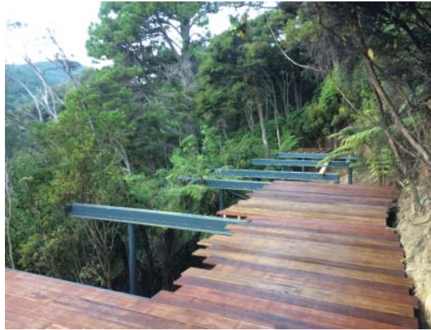
Fig. 29: Boards were left long to be cut with a rail saw later.
