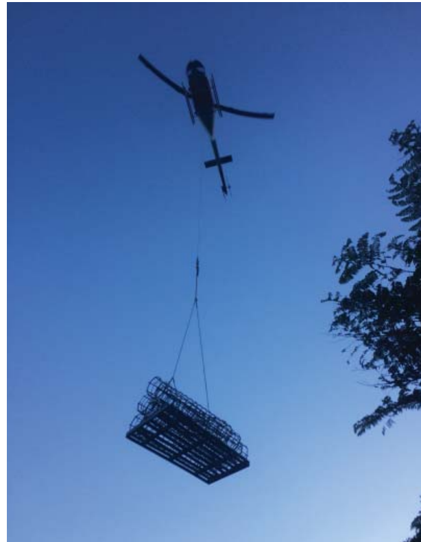
Fig. 15: Pile cages being delivered to the building site.
