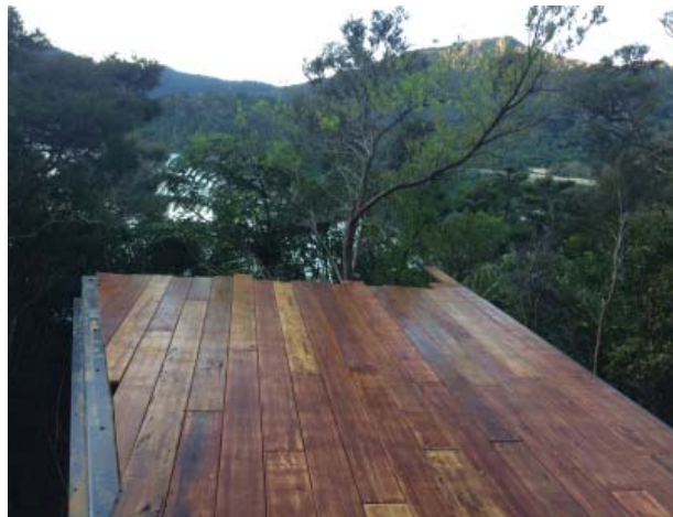
Fig. 31: Decks provided safe working platforms as well as areas to land materials with the helicopter
