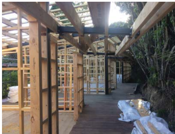
Fig. 61: Wall frames in place, with openings for joinery units.
