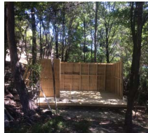
Fig. 105: Standing up the panels.
