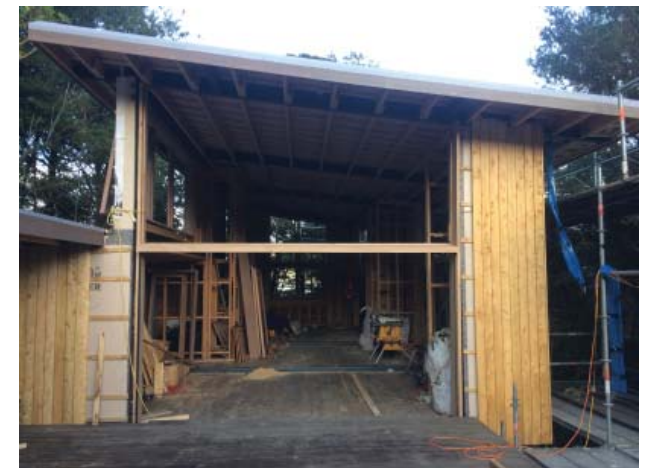
Fig. 92: Cladding into the joinery units.
