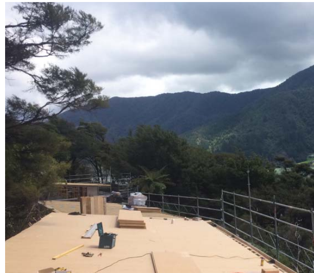
Fig. 56: Fixing 20mm strandboard substrate to purlins in preparation for the T.P.O membrane roof. Note the three different roof planes.
