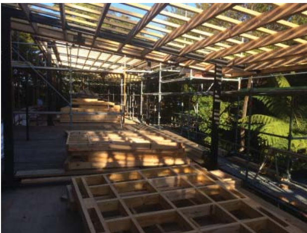
Fig. 60: Wall frames ready to stand up.
