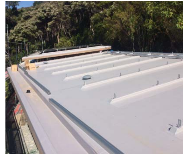
Fig. 57: T.P.O membrane roof with internal gutter, batters provide fixing to mount solar panels.
