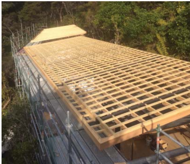
Fig. 55: Purlins at 400 centres, gutter boxed ready for 19mm ply.
