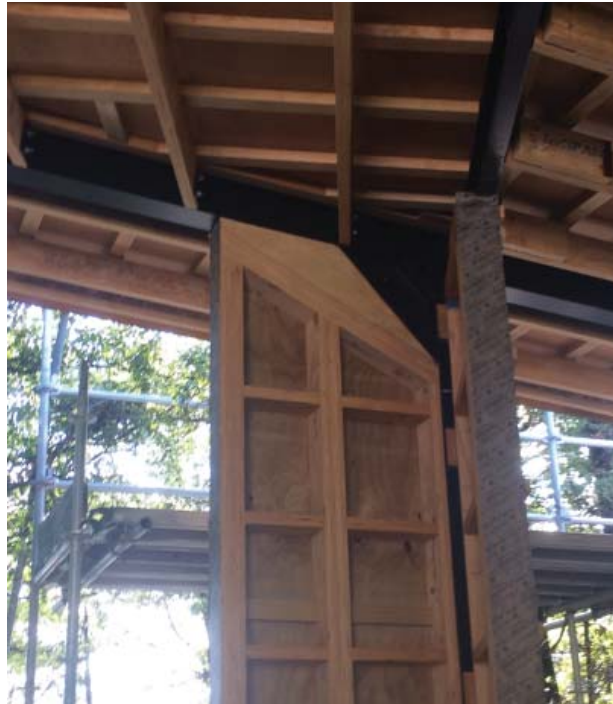
Fig. 58: Blocking around steel to provide fixing for linings.
