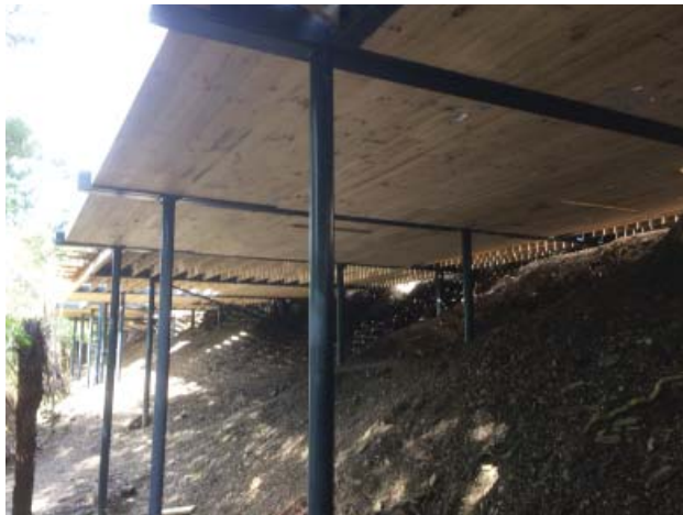
Fig. 44: Panels viewed from below; C.L.T sits on 90x90x6mm EA which is welded to the portal frames.
