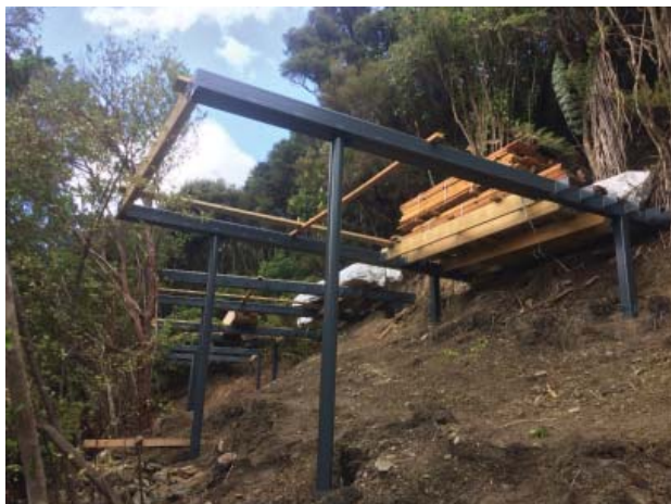
Fig. 26: Sub-floor modules sitting on the pile caps below ground level.
