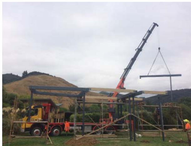
Fig. 22: Modules 1 & 2 in place, module 3 being assembled.
