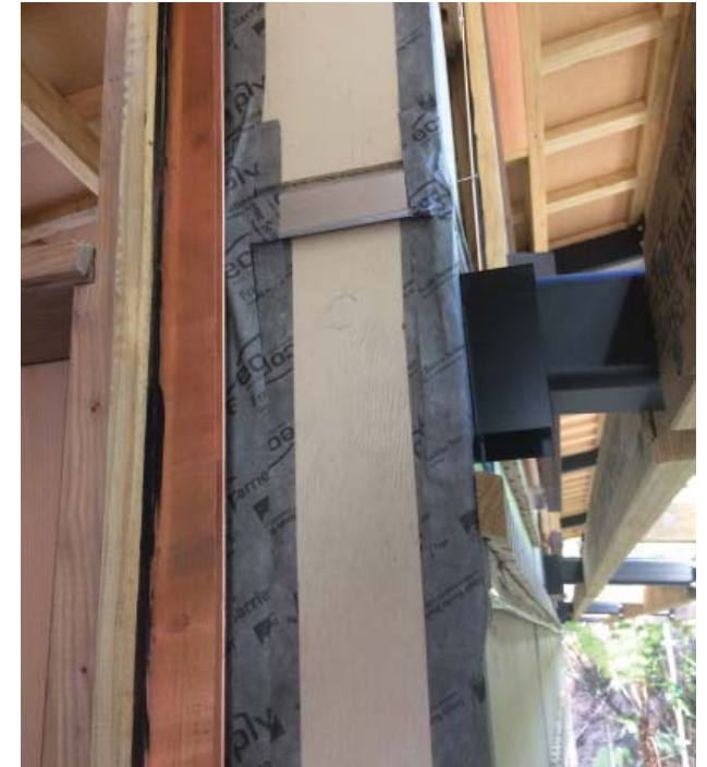
Fig. 59: Busy details: horizontal flashing at ecoply joins, edges taped, joinery opening is taped. Joinery unit is installed followed by jamb flashing with a bead of silicone. Saddle flashings installed where steel protrudes building envelope.
