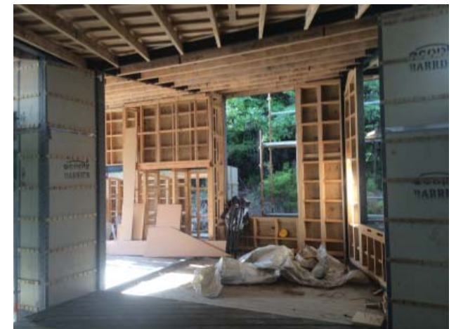
Fig. 62: Wall frames with R.A.B. and cavity battens ready for cladding.
