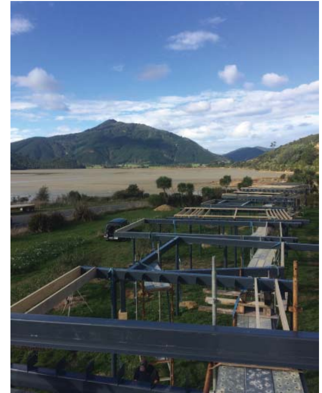
Fig. 20: Modules stopped at lifting points ready for delivery.
