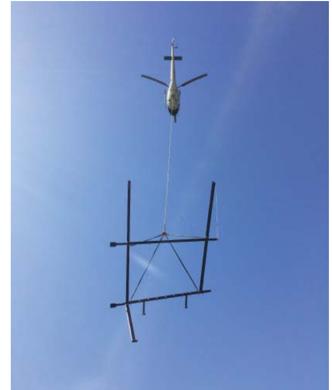
Fig. 50: One legged module being delivered to site.
