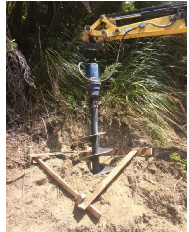
Fig. 10: Drilling each pile, and making sure the auger does not wander.
