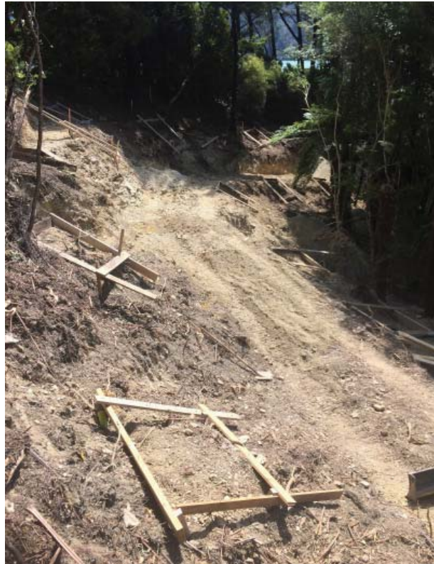
Fig. 9: Individual profiles built around each pile location.
