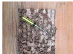
Fig. 33 - 40: 1. Collect offcuts, 2. Cut plugs, 3. Extract plugs, 4. Admire firewood, 5. Pre-drill and countersink fixings, 6. Glue holes, 7. Plug holes, 8. Sand and oil plugs.
