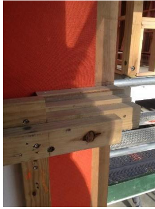
The interstory timber fire break
