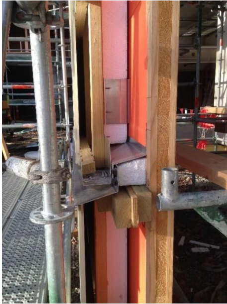
The interstory timber fire break
