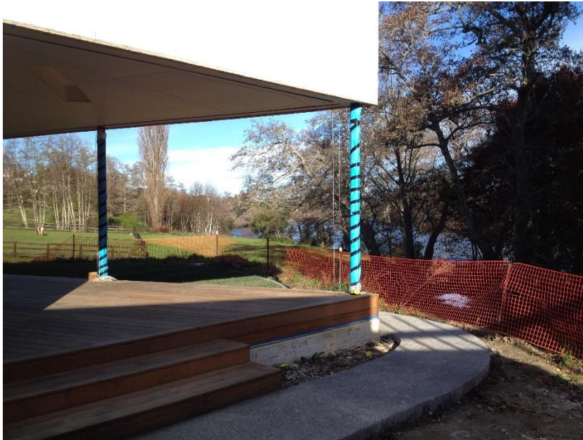
Garapa Decking. Notice also the slots for the weather screen. (Heater yet to be installed in soffit recess)
